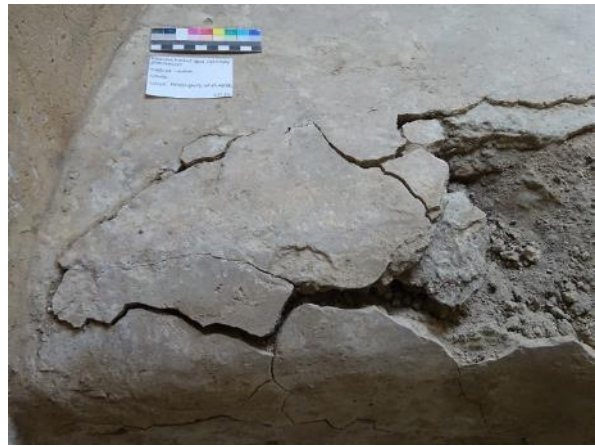
Figure 63: After cleaning and removal of growing plants
