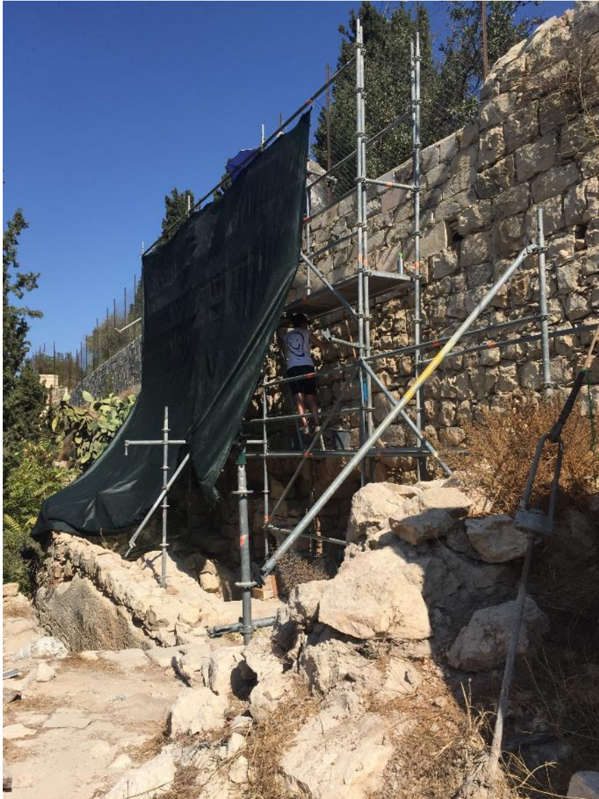
Figure 27: Scaffold in front of cemetery wall (wall A), E. Thierry
