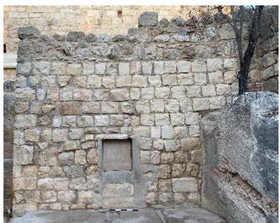
Figure 61: wall D after stabilization measures (2019) and mortar refilling (2021), E. Thierry
