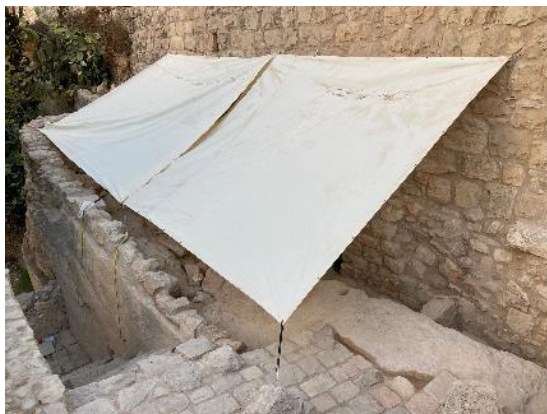
Figure 112: protective rain tarp, 2021
