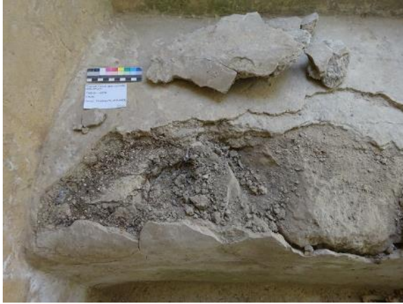
Figure 74: Loose pieces of plaster which are removed to clean the underground
