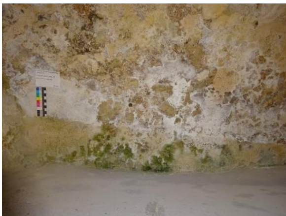
Figure 66: Veils of salt before treatment with a compress
