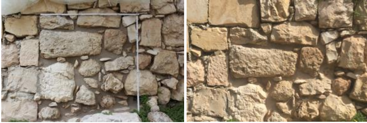
23.01.2018 refilled joints/restored area
