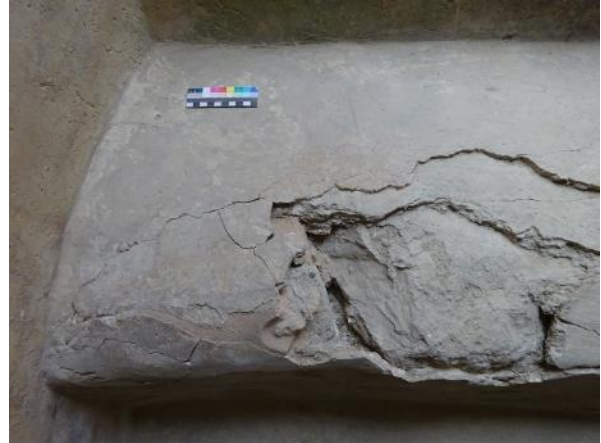
Figure 75: Reapplied pieces of plaster
