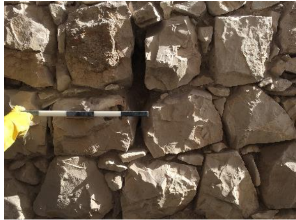
Figure 34: photo documentation area 2: joints scraped out
