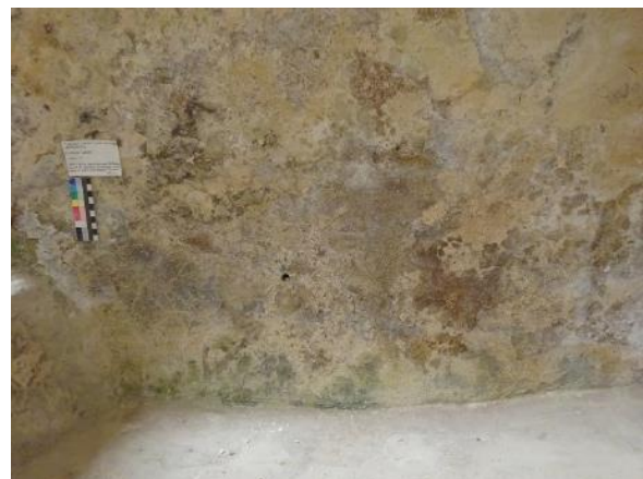
Figure 67: Veils of salt after treatment with a compress
