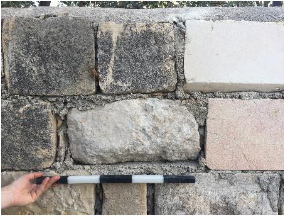
Figure 30: photo documentation area 1: before measure: joints filled with cement mortar
