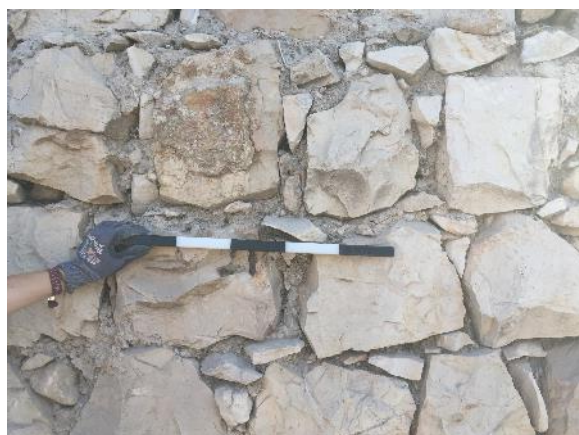
Figure 46: photo documentation area 2: before
