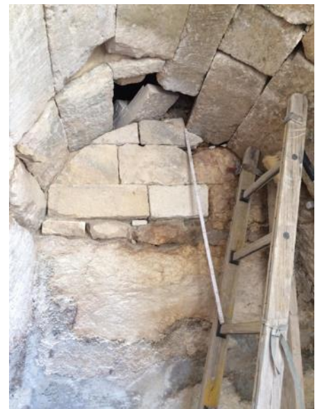
Figure 23: last stone in vault cut in a stepped shape in northwestern Miqveh
