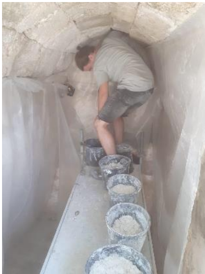
Figure 51: manually filling the hole with lime mortar, 2019
