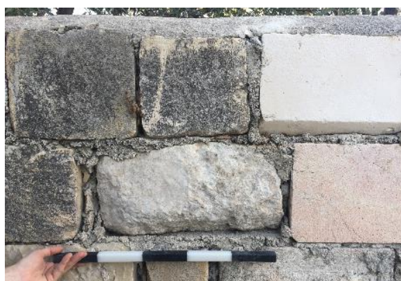
Figure 44: photo documentation area 1: before
