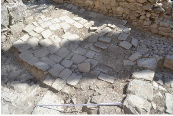
Figure 98: stone tiles before measures, 2016
