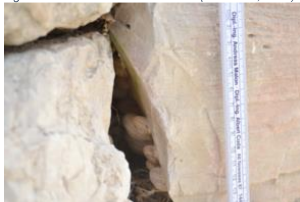
Figure 15: biological colonization in joints, here snails (THIERRY, 2017)
