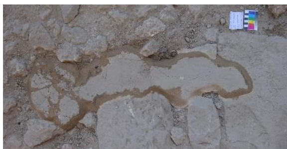
Figure 108: Condition after injections and pointing
