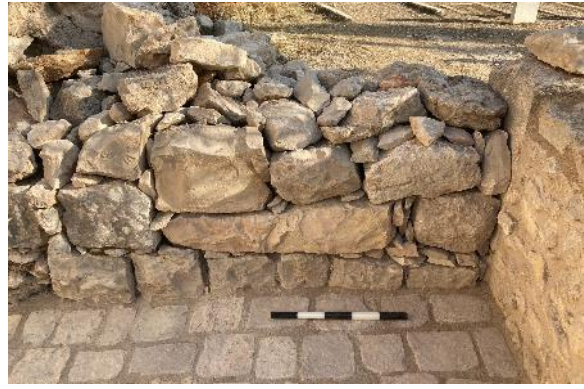
Figure 105: closed access in accordance to the masonry in wall C after measures, 2021
