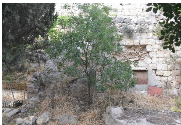
Figure 151: view towards steps and wall D 2016
