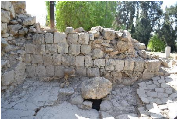
Figure 124: wall C after cleaning but before restoration measures in 2016
