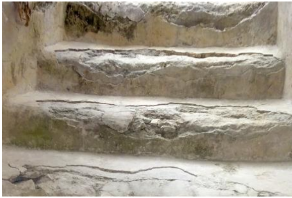
Figure 88: Condition of the stairs after dry cleaning
