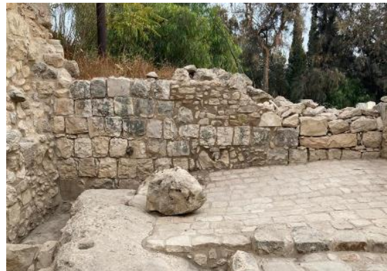
Figure 125: wall C after all measures in 2022
