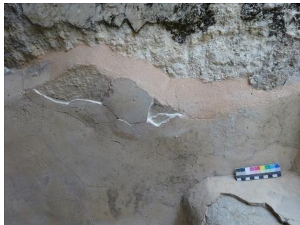
Figure 73: Condition after injections (white material) and partial pointing (orange mortar)
