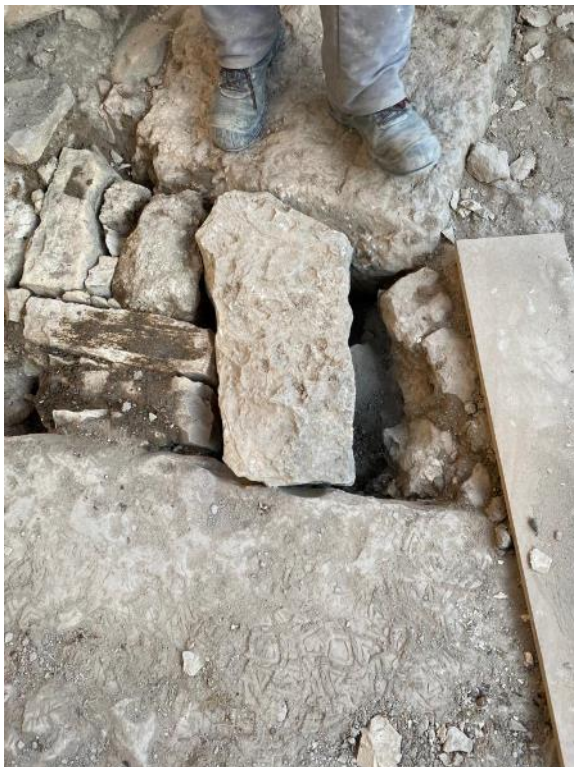
Figure 96: stone with conic shape beared on the rock so structural stability is ensured, 2021
