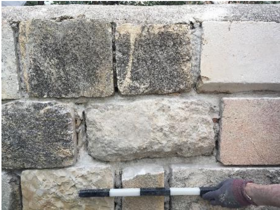
Figure 31: photo documentation area 1: joints scraped out
