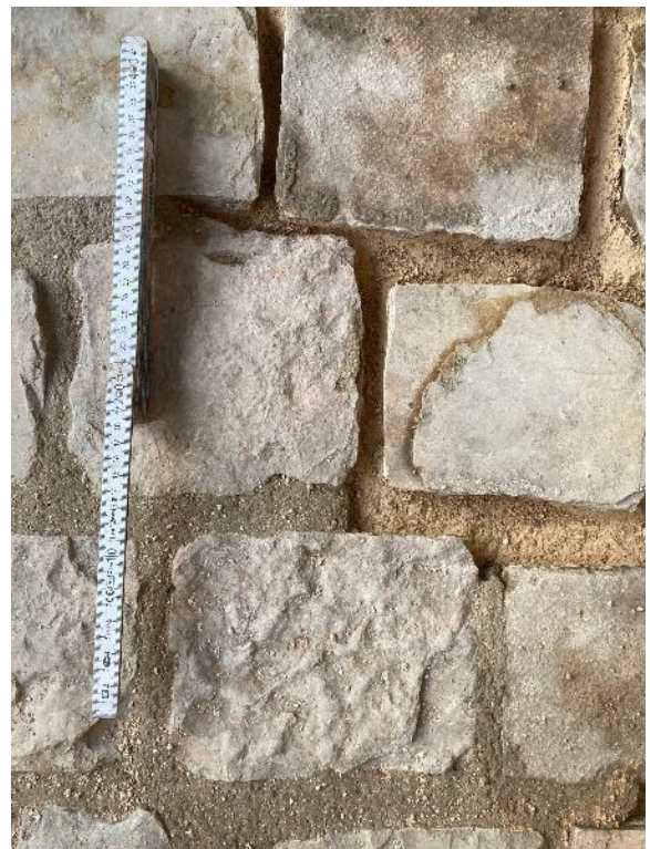
Figure 97: stone tiles in mortar bed; right side: filling non-visible mortar, left side: visible joint mortar, 2021
