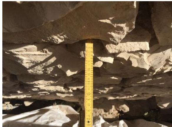
Figure 36: photo documentation area 2: joints scraped out, 5cm depth
