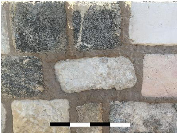
Figure 38: photo documentation area 1: refilling with visible mortar before final smoothing
