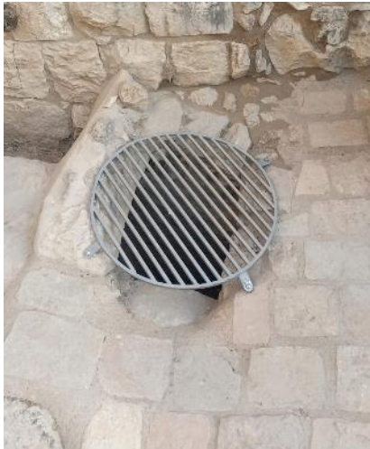
Figure 129: hole to cistern in Miqvot-level with a sustainable long term coverage, 2022
