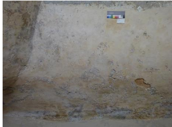
Figure 65: After removal of salt efflorescence
