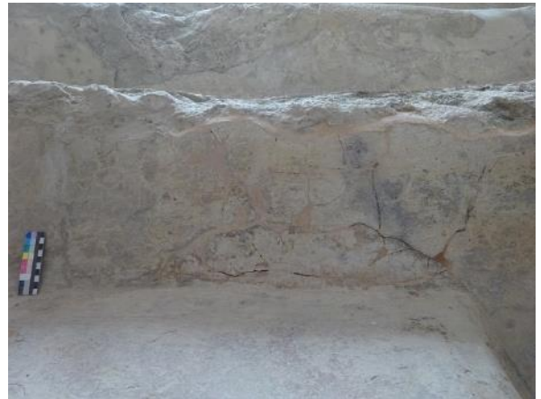
Figure 77: After reapplication of pieces of plaster
