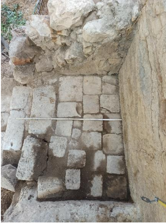
Figure 122: Staircase after cleaning before measures (2022)
