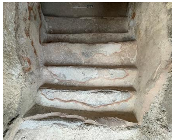
Figure 131: Condition of the stairs after restoration, 2022
