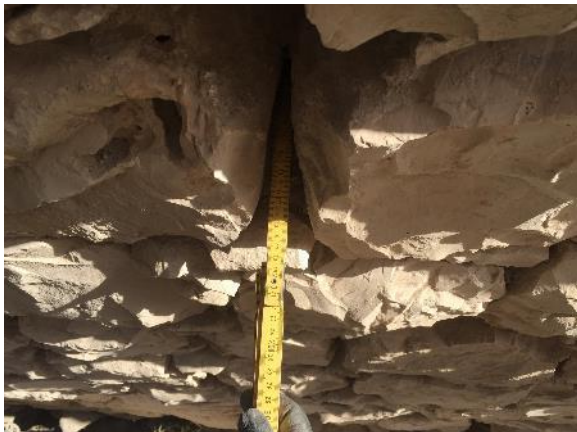
Figure 35: photo documentation area 2: joints scraped out, 15cm depth
