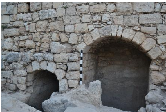
Figure 56: entrances to the Miqvot before measures in 2016
