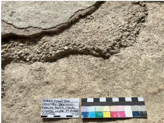
Figure 132: Erosion of the 1st century plaster layer
