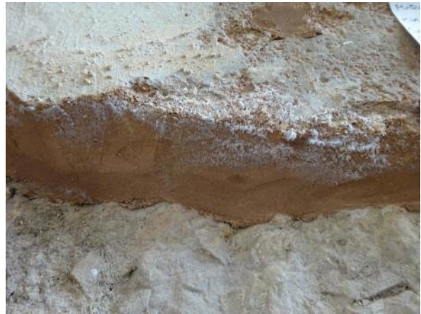
Figure 79: Picture of the new lime based pointing material
