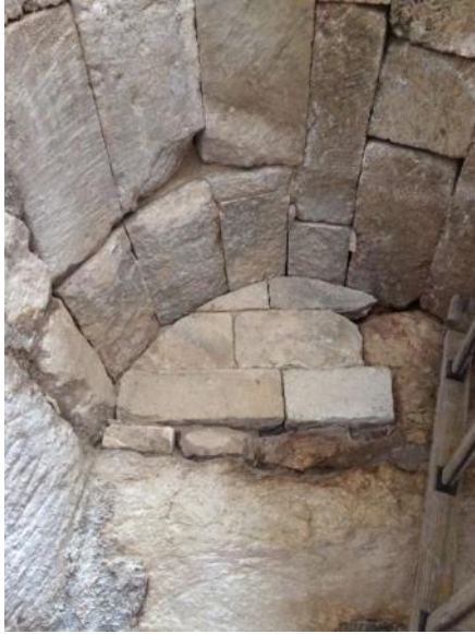
Figure 24: reconstructed vault in original shape, northwestern Miqveh
