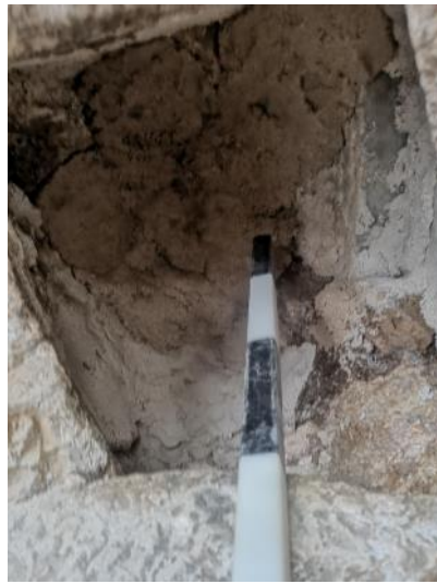
Figure 52: the mortar filled hole, before setting the keystone
