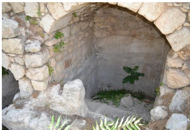
Figure 149: entrance to western miqveh 2016
