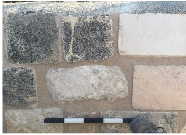
Figure 39: photo documentation area 1: refilling with visible mortar after final smoothing
