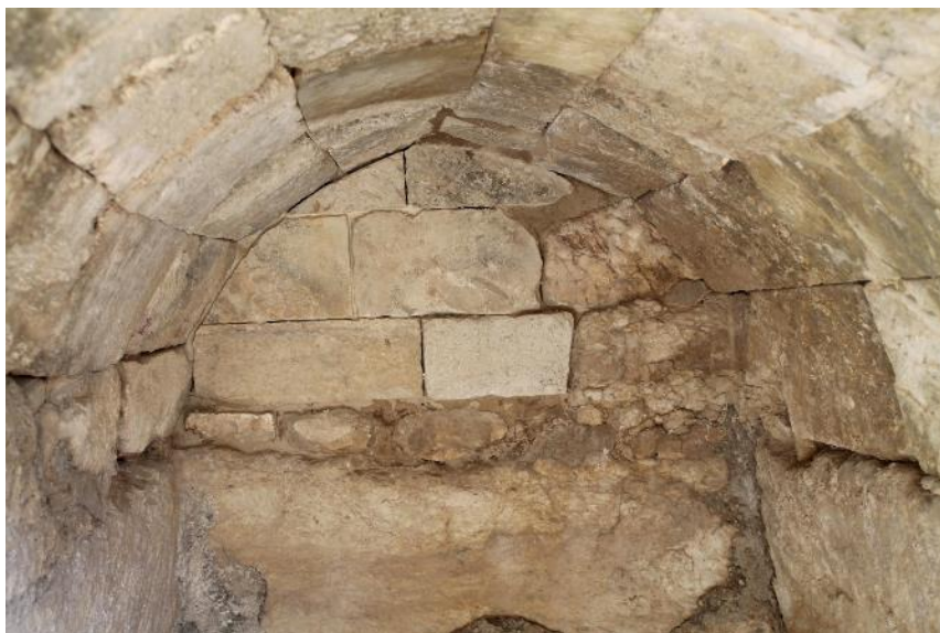
Figure 53: Final restored vault of northwestern Miqveh, 2019
