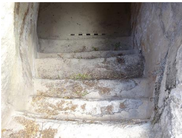
Figure 130: Previous condition of the steps in miqveh 2, 2021
