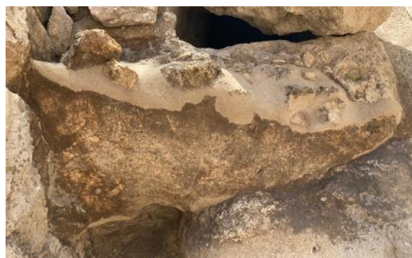
Figure 111: plaster after conservation
