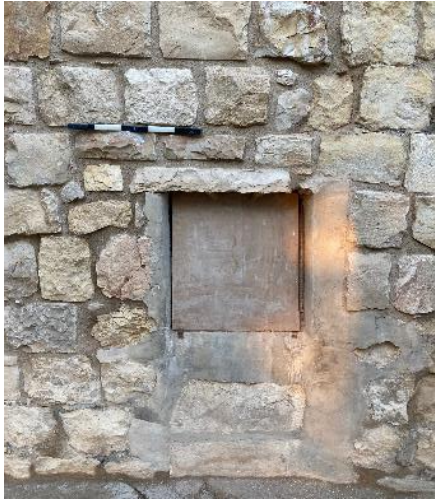
Figure 126: access to cistern with provisory coverage, 2021
