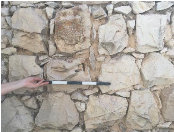
Figure 37: photo documentation area 2: refilling with non-visible mortar
