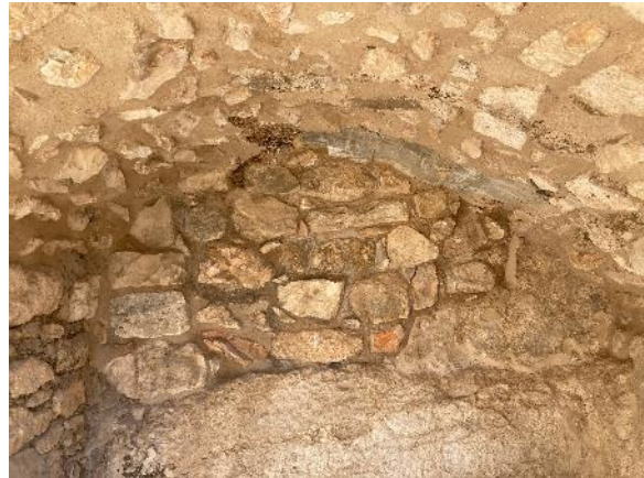
Figure 91: complete restored vault including back wall, 2021
