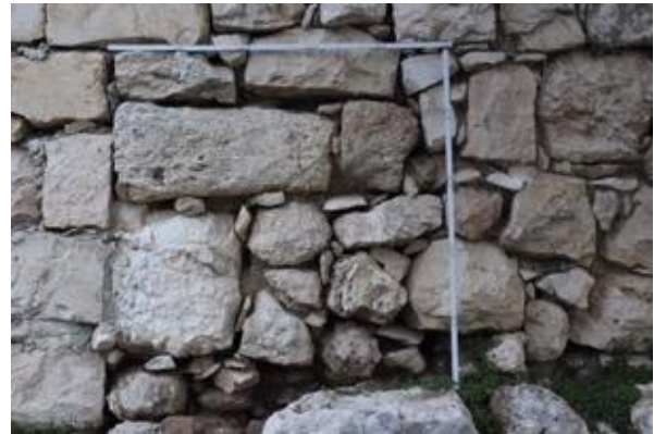
21.01.2018 joints cleaned
