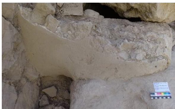
Figure 110: plaster before measures
