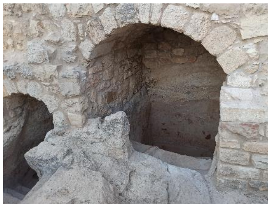
Figure 150: entrance to western miqveh 2022
