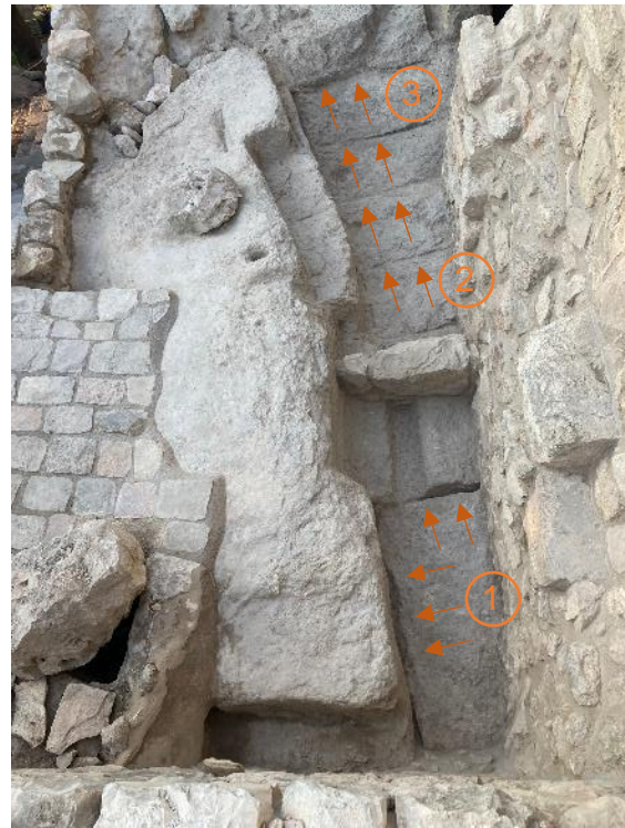
Figure 115: direction of rock hewing according to the stone mason traces, 2021
