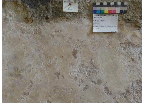
Figure 69: After removal of salt and consolidation
